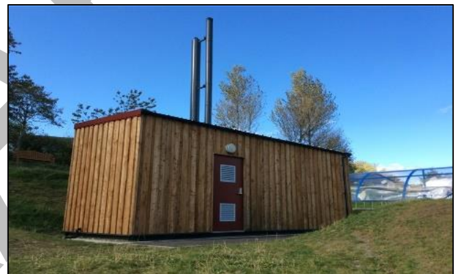
Ardrihaig Primary School biomass boilerhouse
