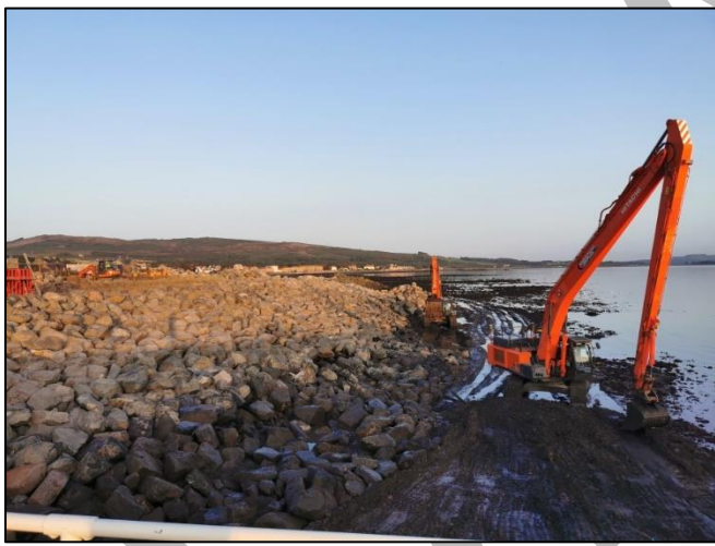
New flood defences being installed at Helensburgh Waterfront, October 2020
