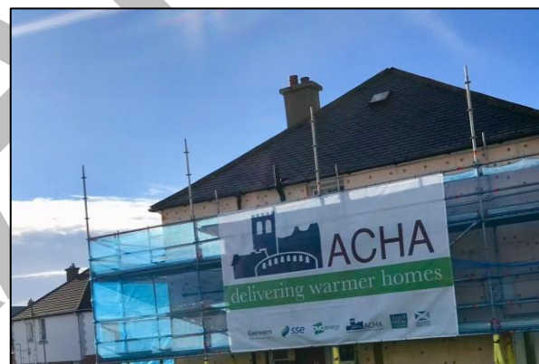
ACHA's External Wall Insulation works in Oban
